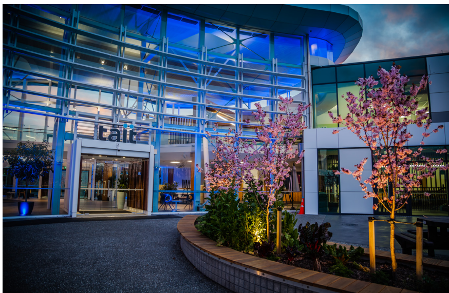
Tait Communications corporate headquarters
